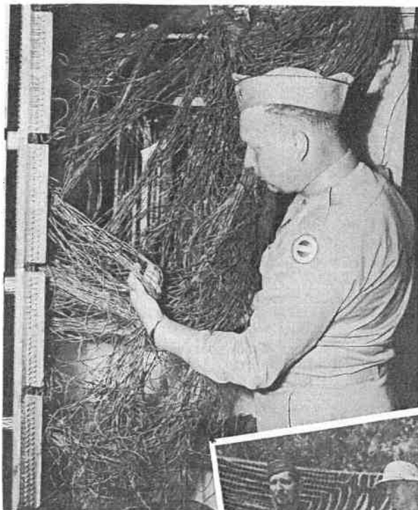
A Typical field communications center, North Africa, June 5, 1943.
